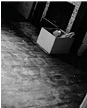
FIGURE 15.3 Visible Dust Indicates Recleaning is Needed
